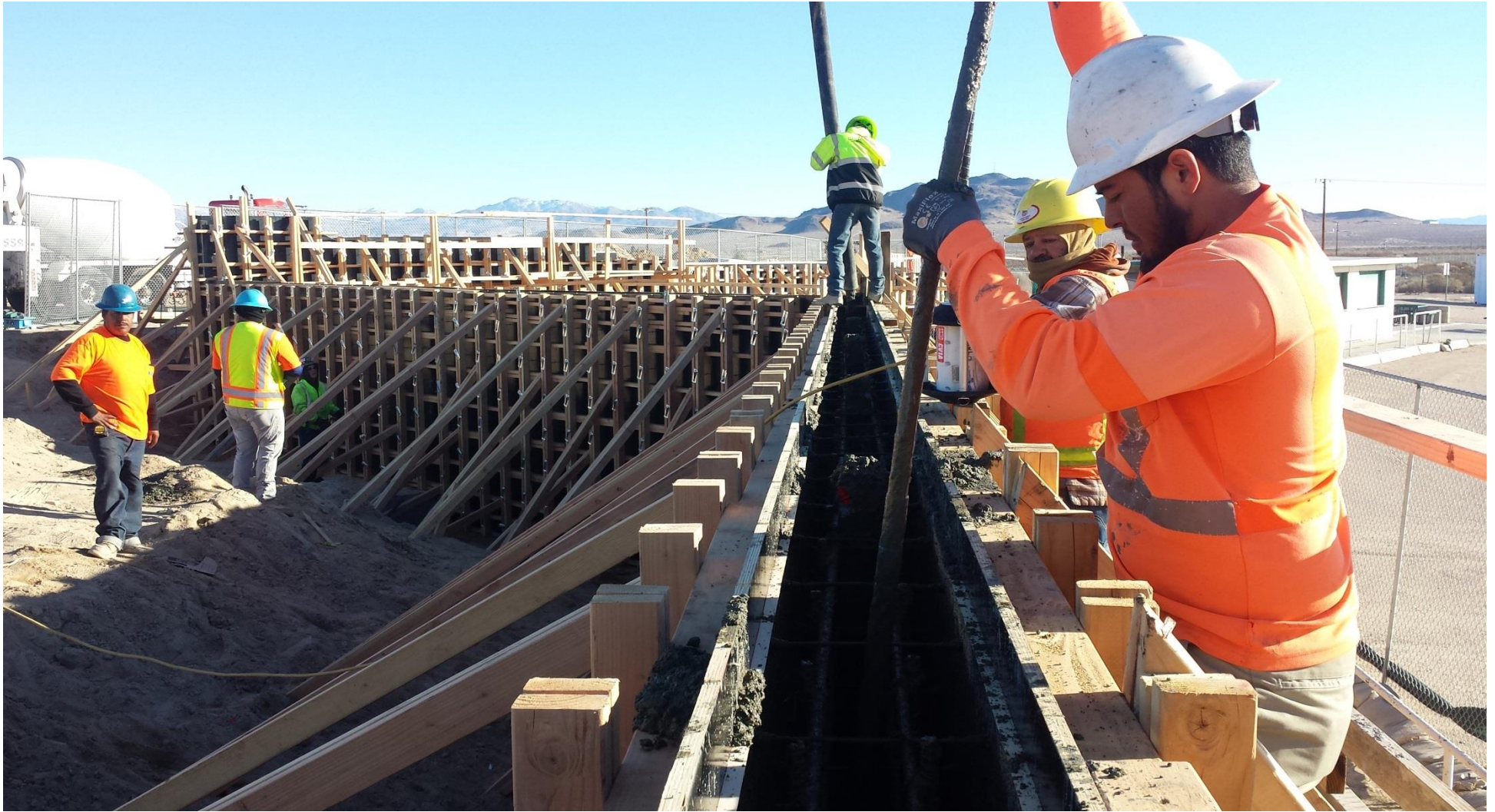
Pouring the patio retaining wall at the New Concessions/Restroom Building
