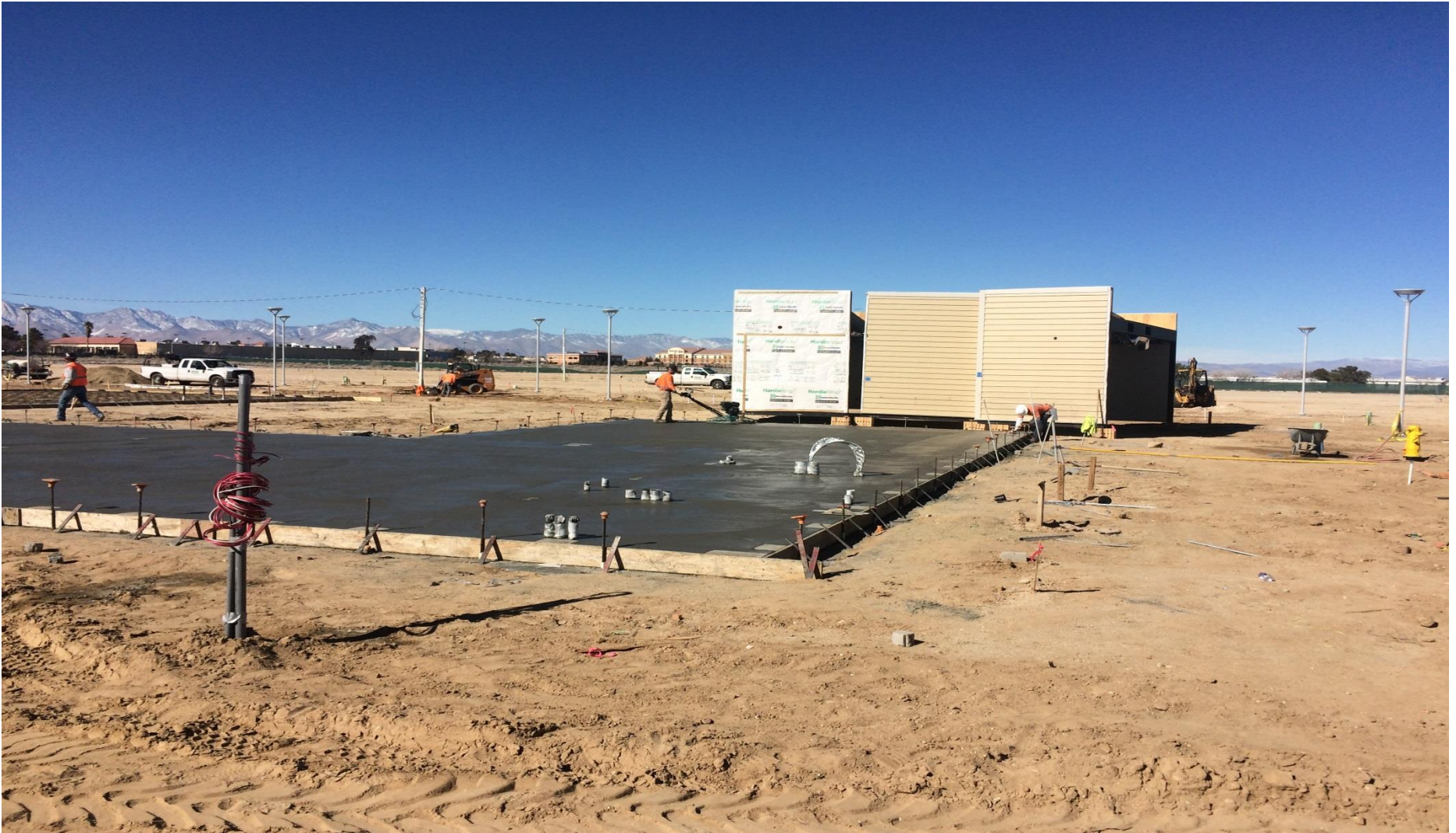
New concrete pad ready to receive classroom modules
